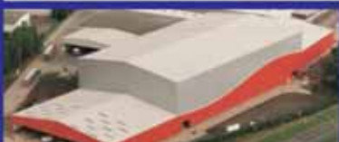
10,000m 2 High Bay warehouse for Coca Cola & Schweppes Beverages Ltd. East Kilbride, Scotland.
