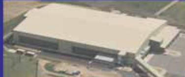
276,000 cubic metre, 100m span ASRS high bay warehouse, with 80 metre conveyor bridge.
