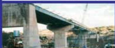
Maphutsaneng Bridge, Mophale Hoek, Mekaling Road, Lesotho, Africa.
