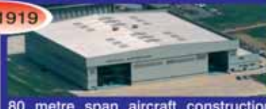
80 metre span aircraft construction hangar for British Aerospace.
